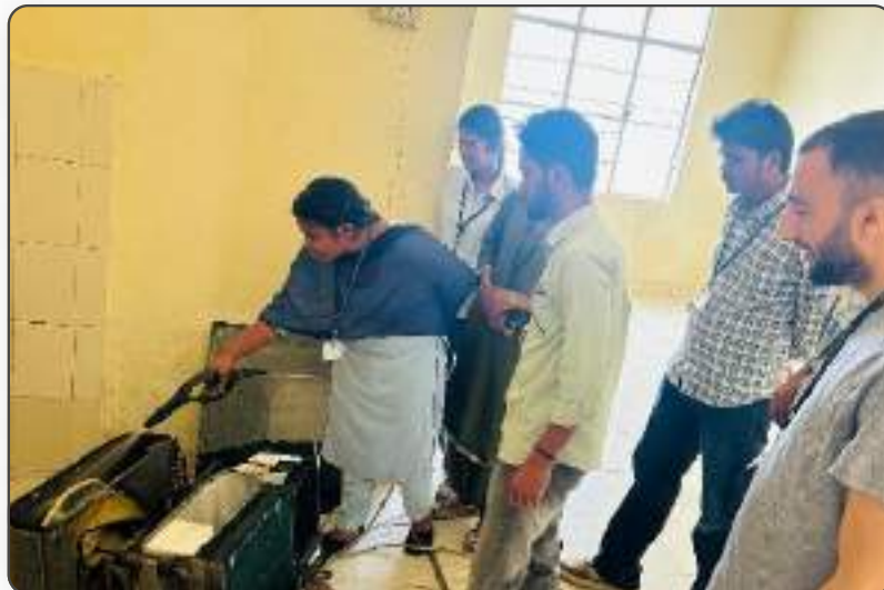
In-house AC Servicing (Institutional Maintenance System)
